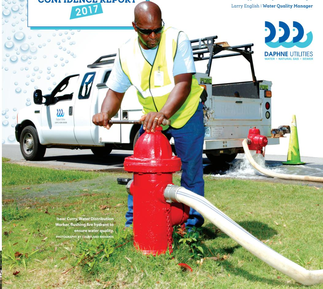
Isaac Curry, Water Distribution Worker, flushing fire hydrant to ensure water quality.
