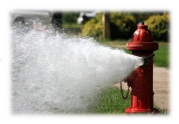
The flushing process is done to remove minerals and sediment that naturally accumulate in water mains over the course of the year. Furthermore, this maintenance allows us to check and record water pressure to ensure the proper operation of the system. Finally, by operating each and every one of the 1,300 fire hydrants in our water distribution system, we ensure each one is properly maintained and available for use in the event of a fire.
